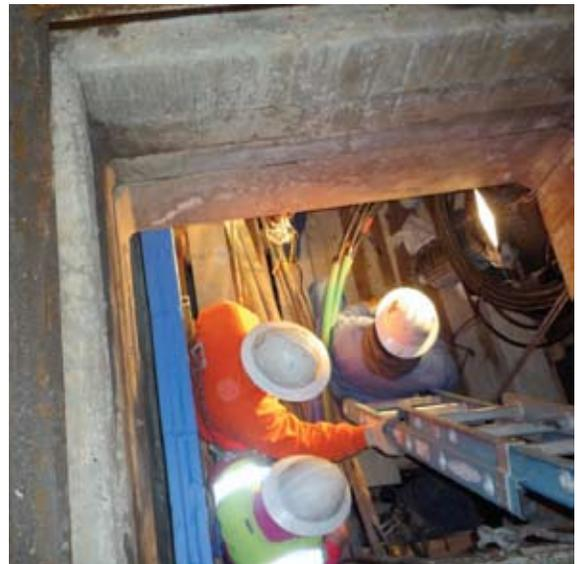
Material for the “vault-in-a-vault” solution was all lowered through the normal access door.
