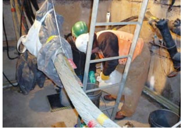
Jeff Kelly, NVE line working foreman, and Vic Camp, Voltek inspector, mixing up grout for the Voltek vault system track.
